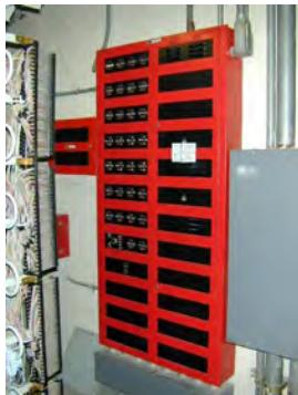
This panel is the control center for the Melville Library fire alarm system. The campus fire marshals are the only ones who have access to this panel in order to reset once it has been activated. It is located in a very secure area.
