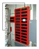
This panel is the control center for the Melville Library fire alarm system. The campus fire marshals are the only ones who have access to this panel in order to reset once it has been activated. It is located in a very secure area of the
